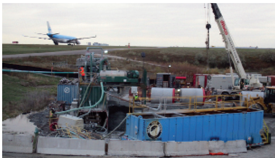
Once operational, the new sewer at Lester B. Pearson International Airport in Toronto will provide added capacity running in parallel with the existing 1,650 mm sewer already under operation. The Region of Peel will have the ability to use either or both of the twinned sewers at any time.
