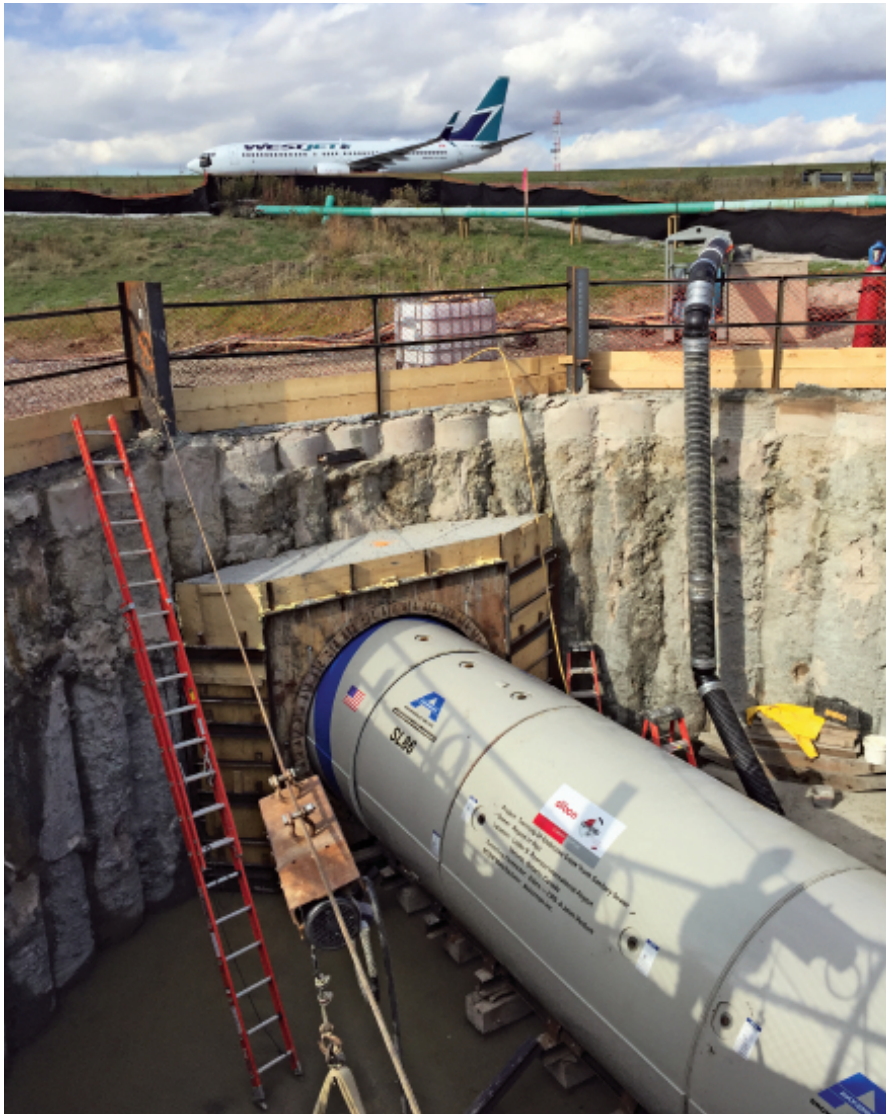
CRS/Dibco recently completed a project involving the construction of approximately 576 m (1,890 ft) of 1,800 mm (70.8 in.) internal diameter sewer underneath Runway 23 and Taxiways J and H at Pearson International Airport in Toronto.
