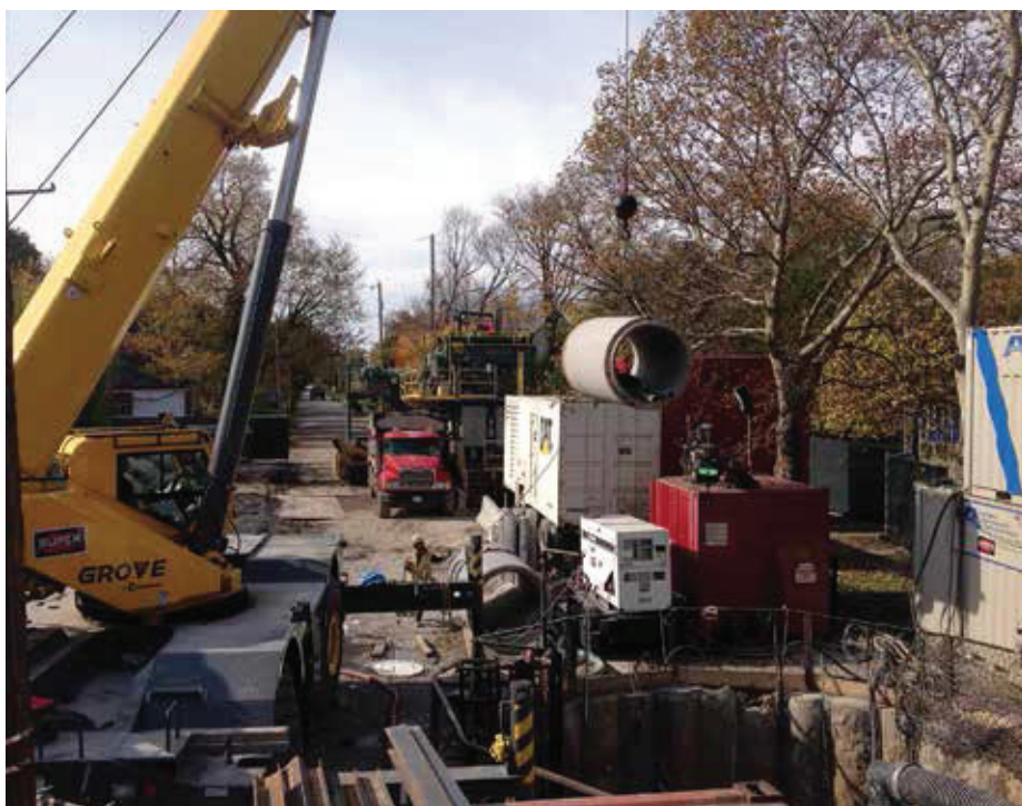
The DWIRS project involves ongoing works with an above ground contractor.
