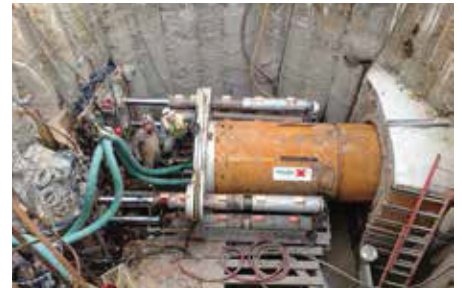
The launch pit for the microtunnelling application during the Dugway West Interceptor Relief Sewer project.
