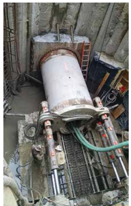
An aerial view of the MTBM launch pit.
