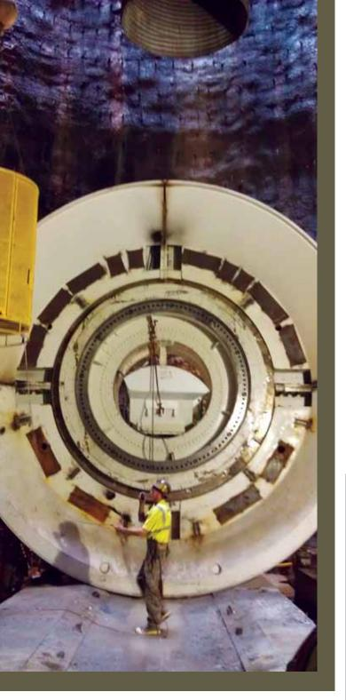
as crews began preparing for the arrival of the tunnel boring machine. Crews are using a refurbished Robbins double-shield TBM with a new cutterhead.
